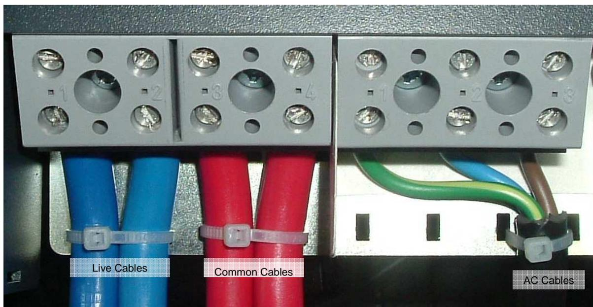
**Fig 3.** AC and DC cable strain relief
