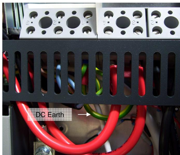
**Fig. 2** System DC Earth connection
